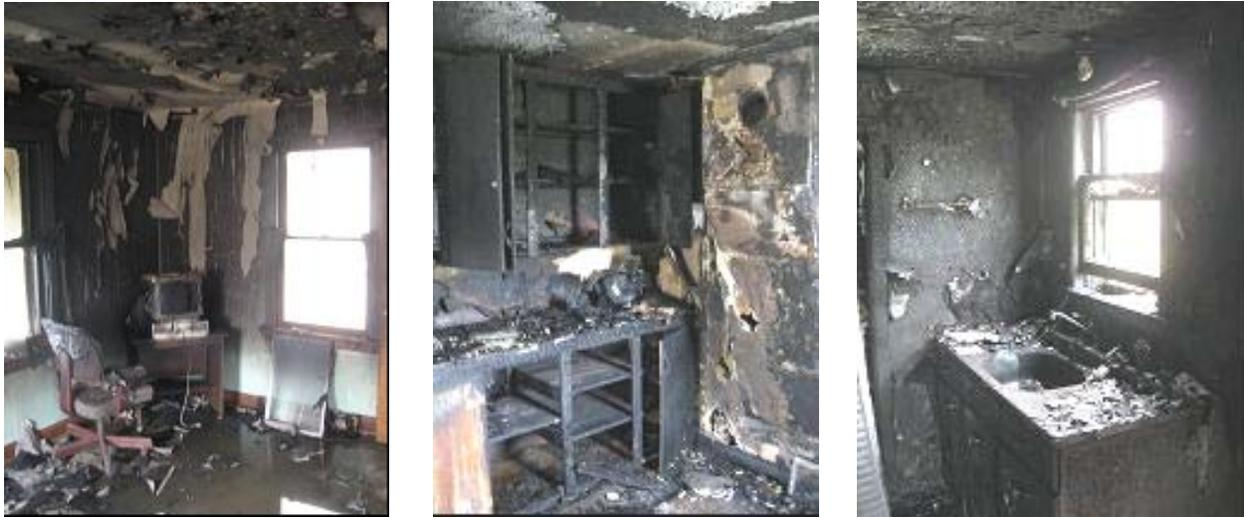
**Figure 5-10: Kitchen after the controlled field fire event.**
