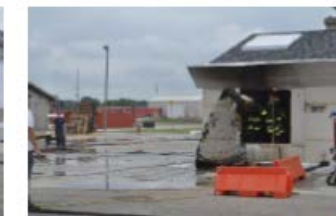
Overhaul Teams remove debris and drywall from fire rooms
